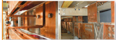
▶ ELEKTROLYSIS: BUSBARS
