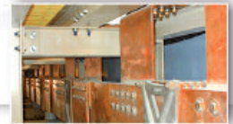
▶ ELEKTROLYSIS: BUSBARS
